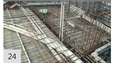
Installation of Electrical and Plumbing components
