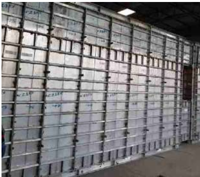
Setting of Wall Panel
