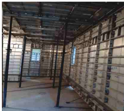
Fixing of Waler in Wall
