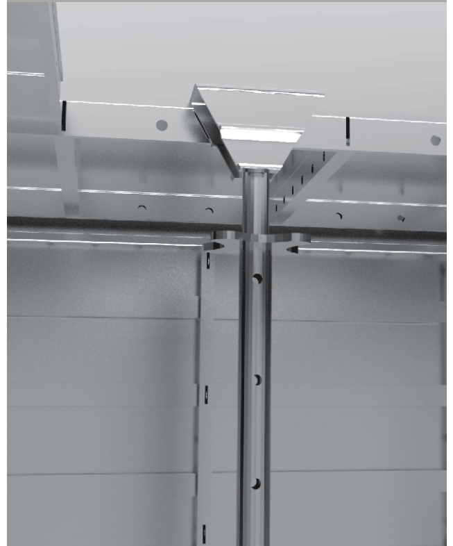
Dismantling of Slab Panel
