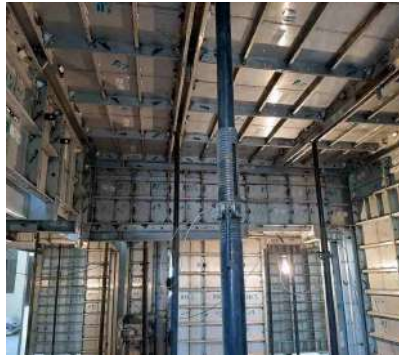
Setting of Slab Panel
