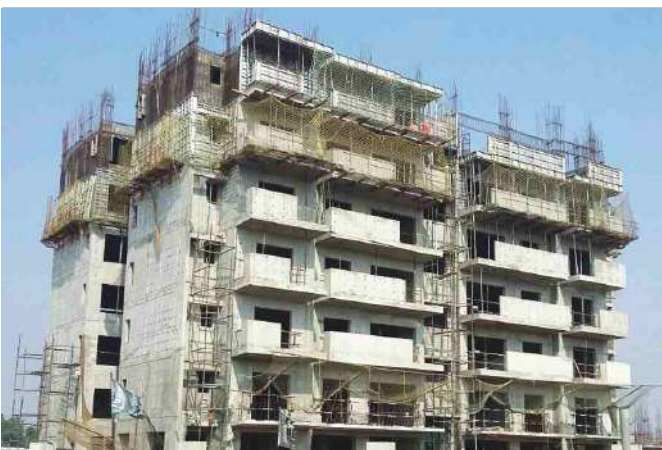
Project - TATA Housing - New Heaven - Bahadurgarh
