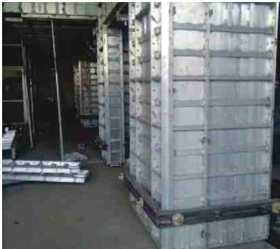
Fixing of Waler in Column
