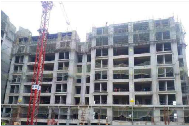
Project - Sai Construction- Godrej Nurture, Bangalore
