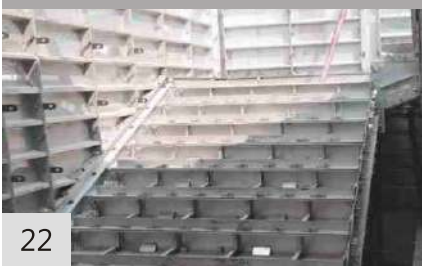
Setting of Staircase
