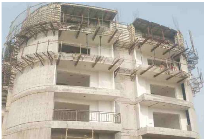
Project - Rishita - Mulberry Heights, Lucknow
