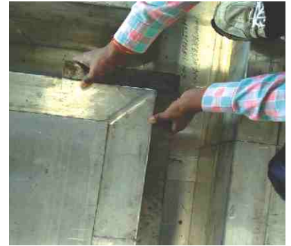
Checking of Slab Corner
