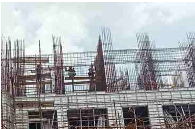
Project - Sobha- Dream Heights, Gujarat
