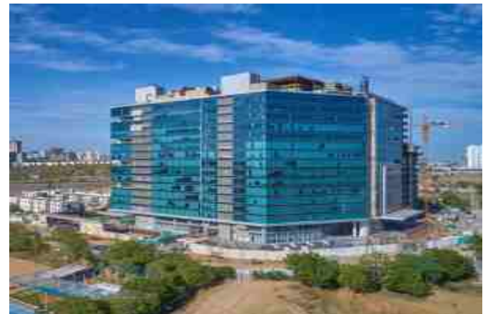
Project - Metro Buildwell - GAR Laxmi Infobahn, Hyderabad
