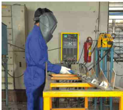
MIG Welding of Special Profile
