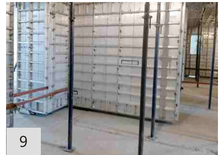
Setting of Slab Panel
