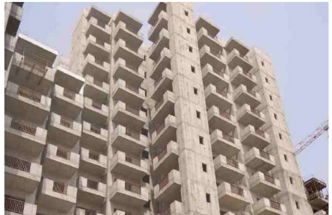
Project - GLS Infra-Arawali homes, Gurugram
