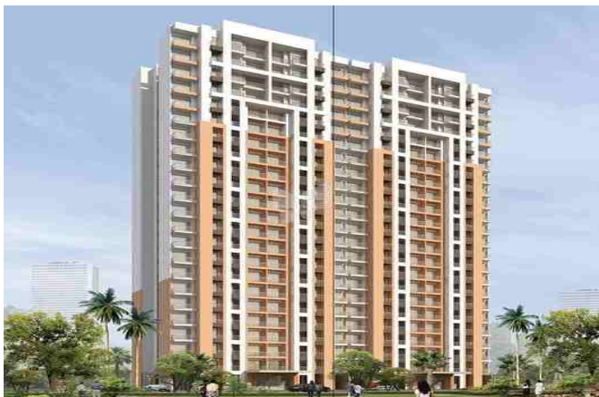
Project - Lodha Casa Plava II - Mumbai
