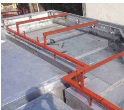
Fixing and Alignment of Balcony
