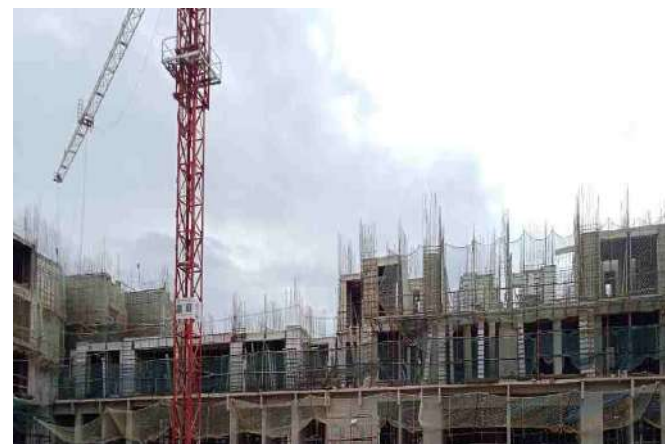
Project - Sai Construction- Godrej Nurture, Bangalore
