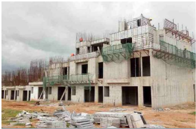
Project - Assetz - Earth & Essence, Bangalore
