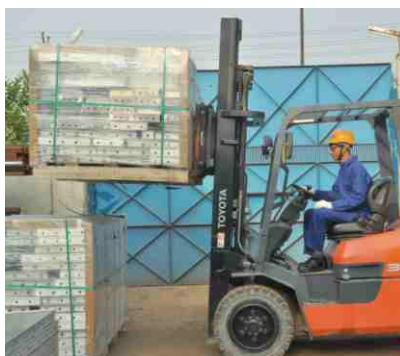
Stacking of Materials
