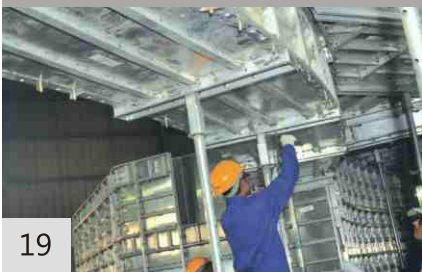
Setting of beam bottom
