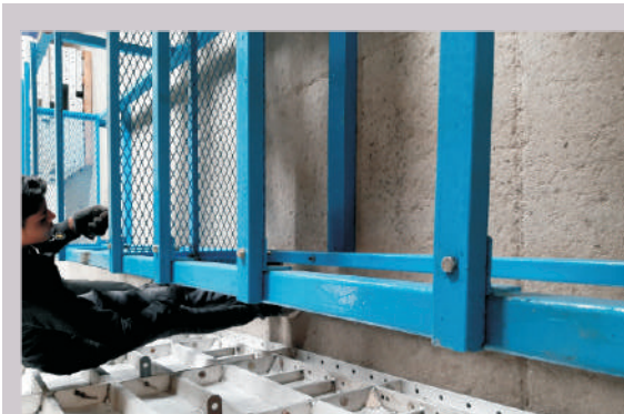
Fixing of Safety Grill
