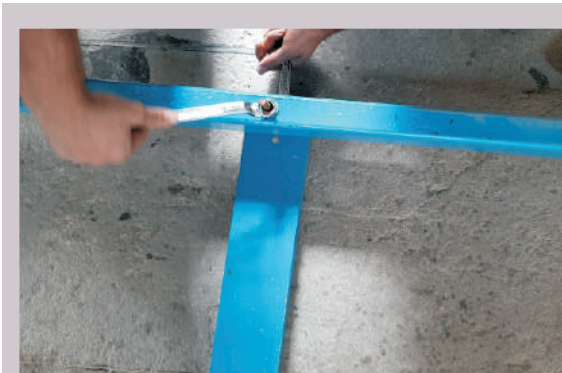
Fixing of Frame
