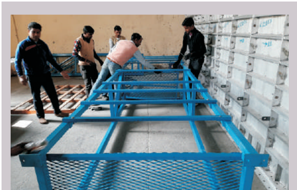
Assembling of Wind Screen
