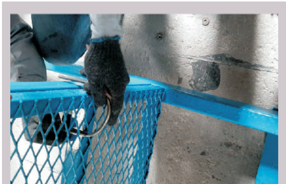
Fixing of Platform
