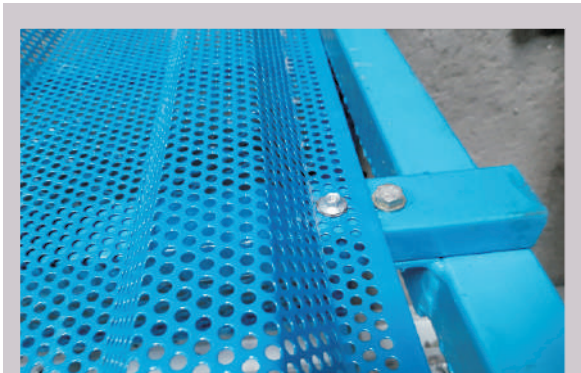
Fixing of Perforated Sheet
