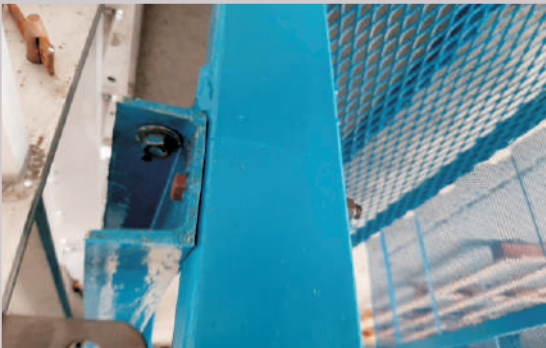
Fixing of Hanging Channel
